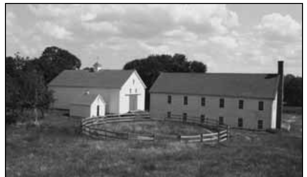
Wright-Locke-Hamilton Farm – 1915 Squash House (right), c. 1900 Ice House (left front), and 1827 barn (left rear). Courtesy of Mark Flannery.
